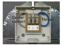
**Do NOT connect any of the ballast outputs to the middle (ground) terminal.** Connecting the ground wire to the center terminal only provides protection when the ballast is also plugged into a grounded receptacle with a grounded cord and plug. This is the recommended way of installation.
